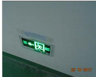
Photo of the inside of the main production hall Evacuation sign.JPG
